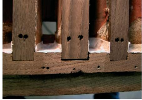
Figure 37. Channels in the bar frame. The small holes are for the pallet guide pins.
