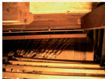
**Figure 9. Pneumatic action under the windchest.**
