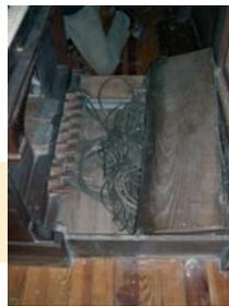
**Figure 8. Plastic pneumatic tubing at the 1934 console.**
